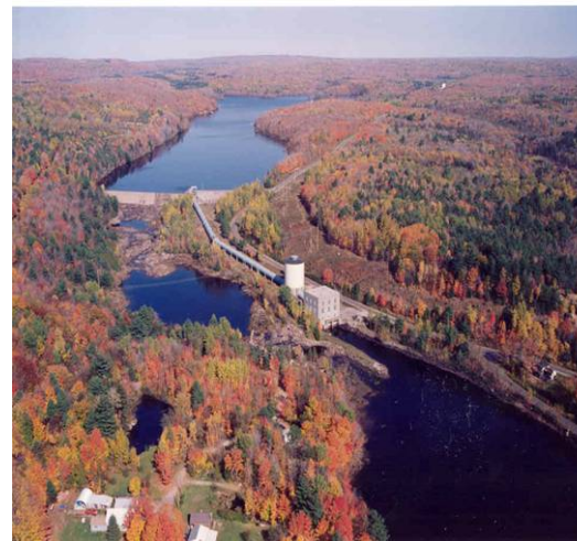
South Colton Hydropower Plant
